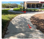
Further grinding correction location showing height differential.
